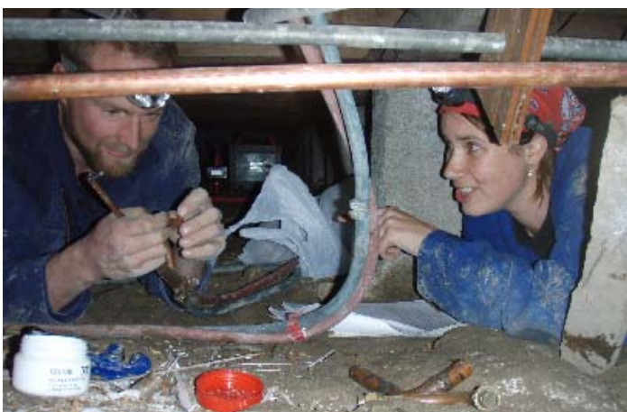
While Pete was visiting us he helped Dad with a job. Here is a picture of us under the house finishing off the job. In front of me are, "The Questions," lying there with me in the mud. We took every opportunity to discuss them.
